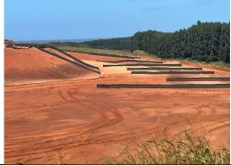
Sediment fences erected at C-extension to reduce windblown dust.
