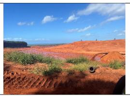
Filling of mined out areas in C-extension. Once shaped to the final profile these areas will be rehabilitated
