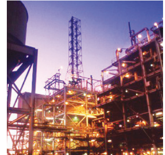
Kemerton Plant 869 Marriott Road Kemerton Industrial Park, Australia
