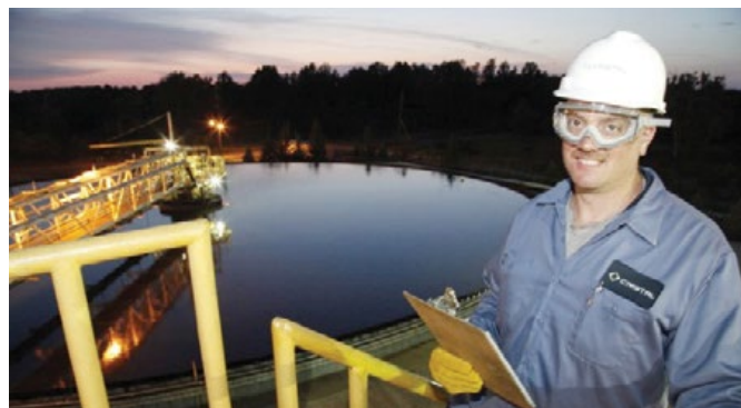
Wastewater at Ashtabula complex is treated prior to discharge.
