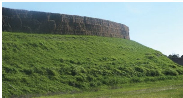
Noise control structures at Wonnerup
